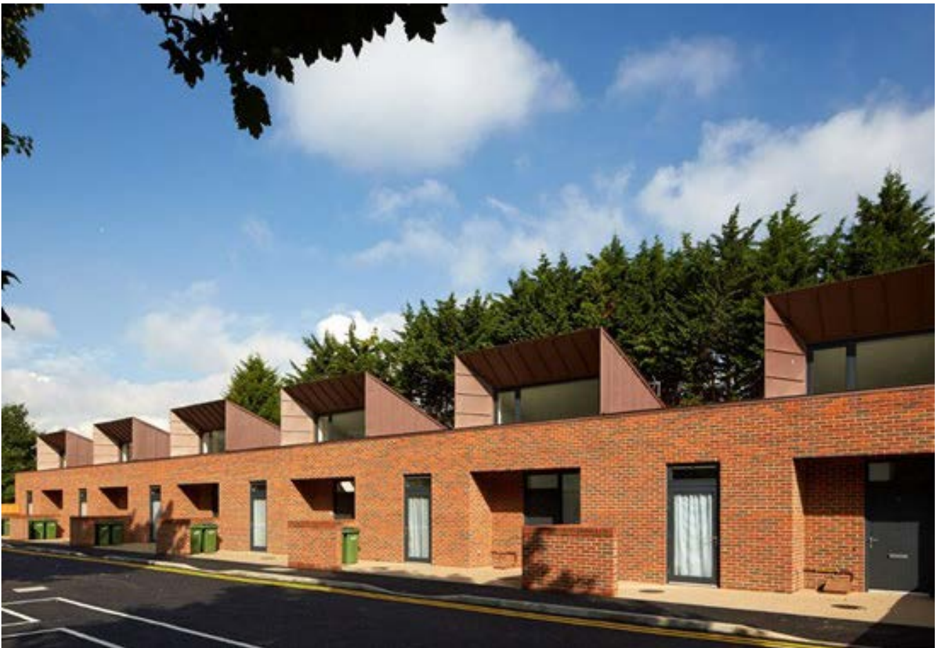
Figure 30: the unique, space efficient design of Ravens Way Houses is very apparent from the front of the development, which overlooks the front courtyard. The approach to fenestration makes the most of available space.
