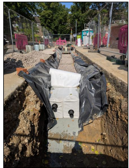
Wellesley Road hydrorock installation
