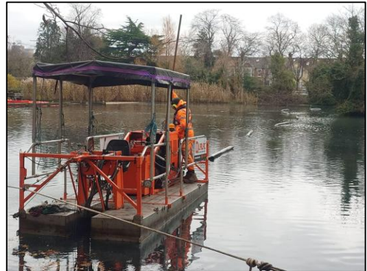
South Park Lake dredging
