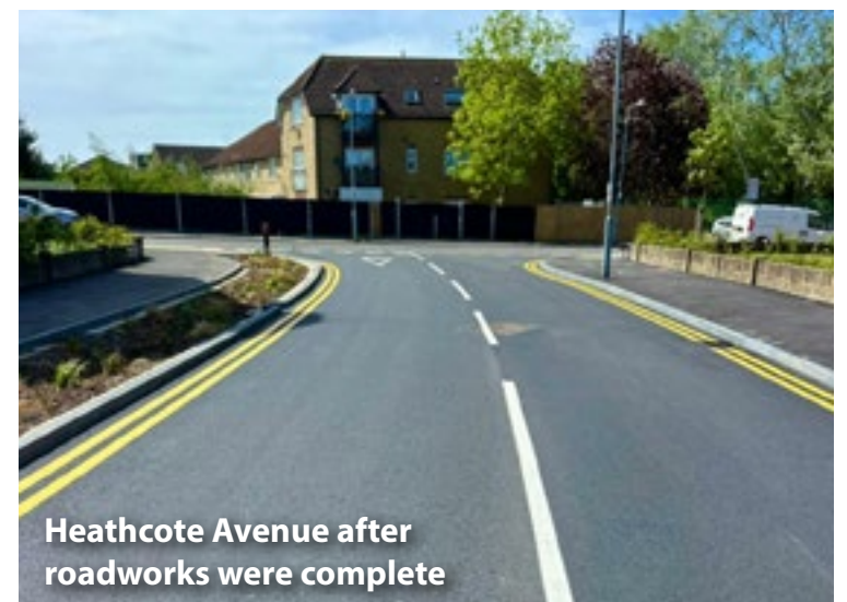
Works on Heathcote Avenue, in Clayhall
