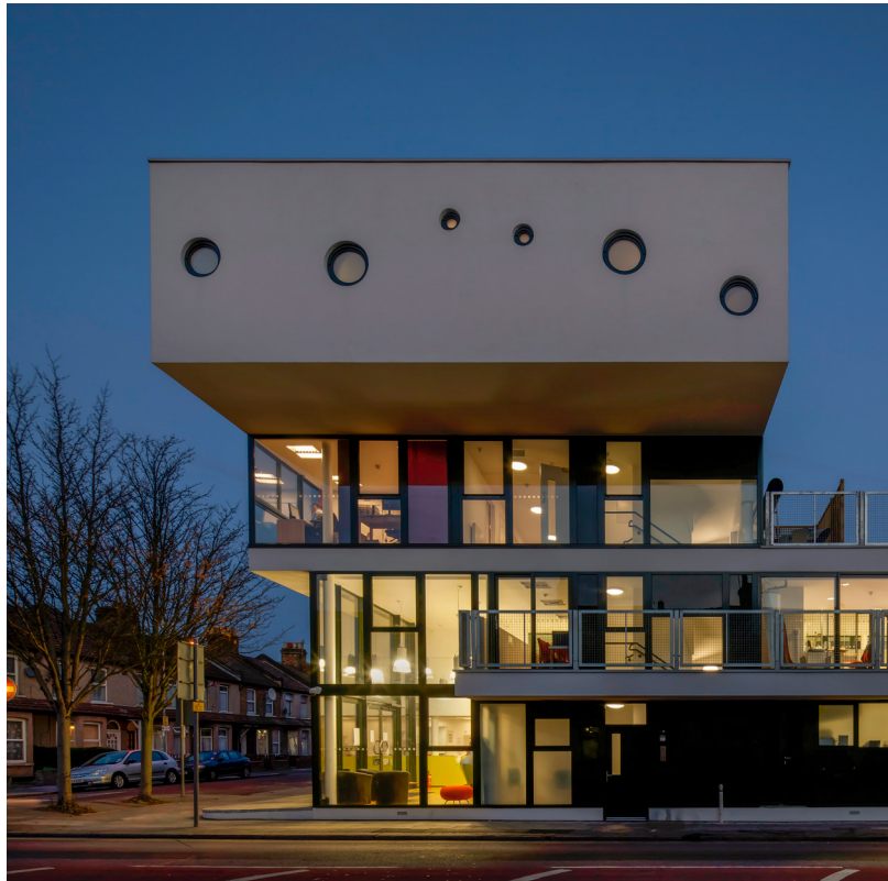
Redbridge Welcome Centre, Peter Barber Architects © Morley von Sternberg
