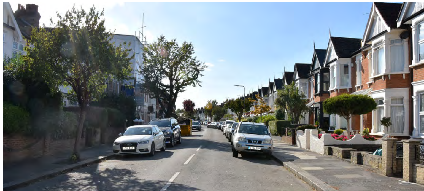
View west along Harpenden Road from its eastern end showing the negative impact on collective character arising from individual missing architectural details (such as a missing gable finial)
