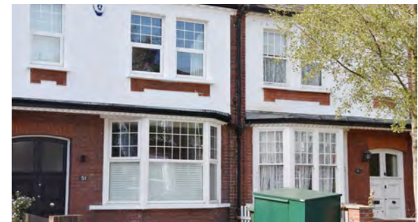
Examples of exposed brick and roughcast wall coverings within the Conservation Area
