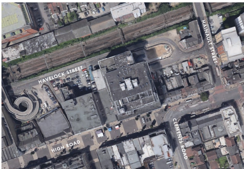
The existing site at Havelock Street
