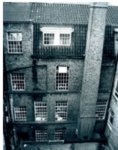
Kentish Town Building prior to refurbishment
