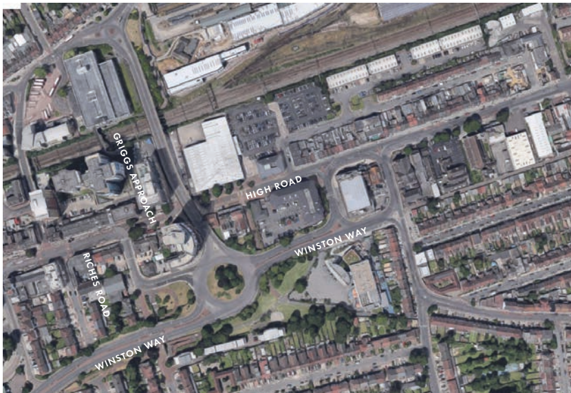
The existing area around the Winston Way roundabout
