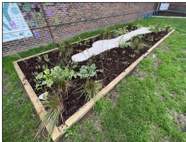
SuDS planter and rain garden installed at Caterham High School
