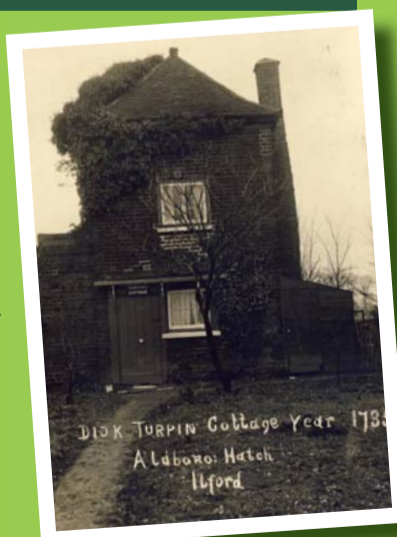
Aldborough Hall, (former garden gazebo)
