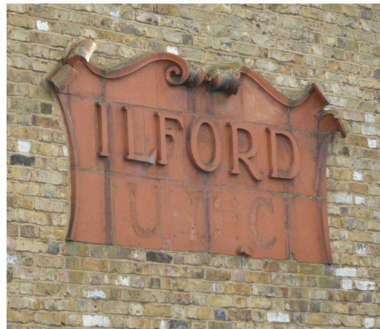
Former Trolleybus Depot, Ilford © Chris Walker / Flickr
