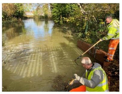
Figure 3-5 Water level at the trash screen while being cleared by Redbridge contractors. Source: EA
