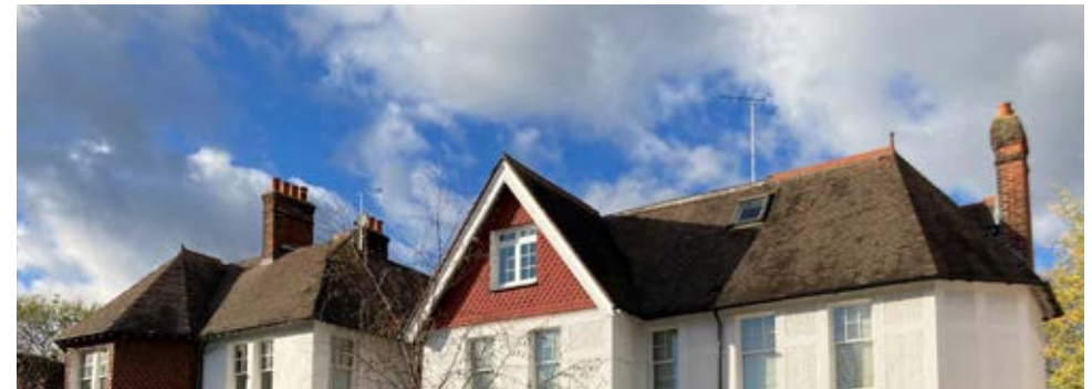
Figure 37 Varying roof styles within the character area
