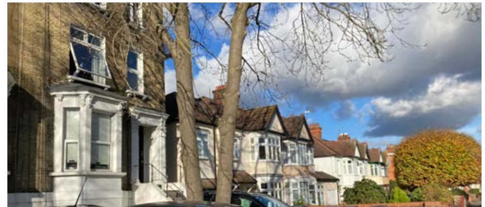
Figure 22 Transition from Grosvenor Road (west) to Grosvenor Road (east)
