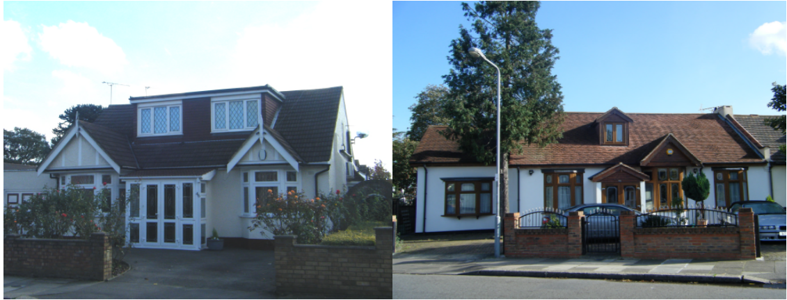
L/ harmful large box dormer and porch. R/ unsympathetic window replacements in wood-effect PVCu and urban character 'brick and railing' front boundary treatment.
