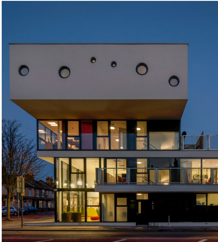
Redbridge Welcome Centre, Peter Barber Architects © Morley von Sternberg
