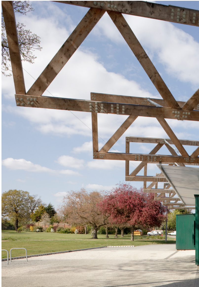
Ray Park Visitor Centre, Sarah Wigglesworth Architects © Mark Hadden
