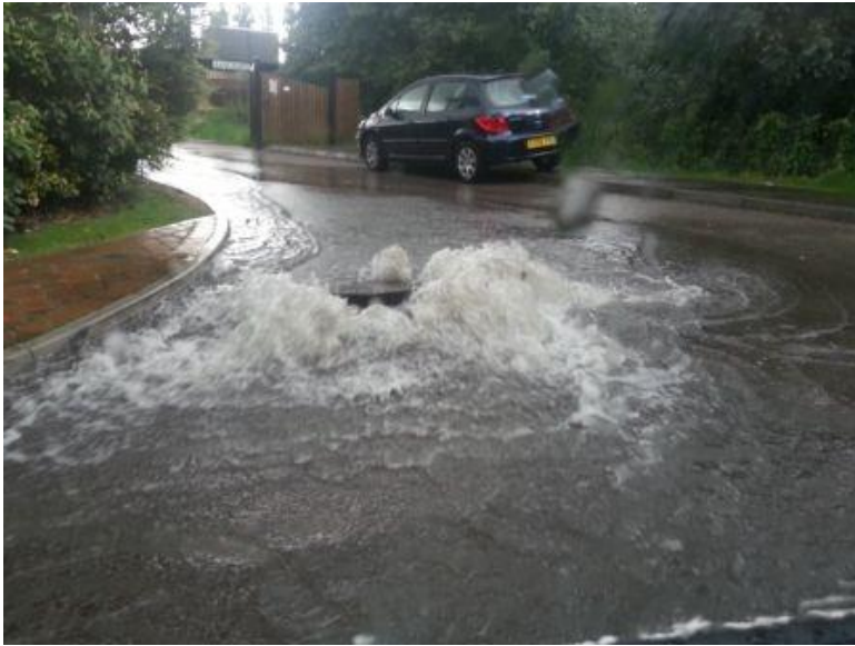
Figure 3.3: Photograph of an overflowing manhole due to overcapacity in the Thames Water sewer
