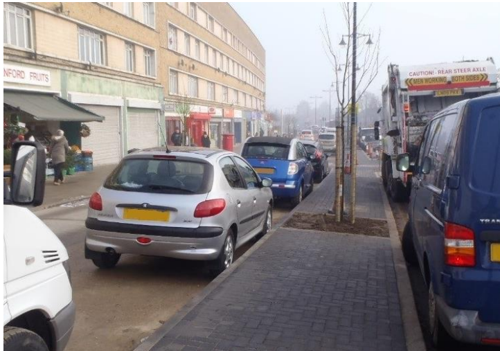
Figure 9.1: Photograph of a Manford Way tree pit which incorporates a soakaway and gully connection
