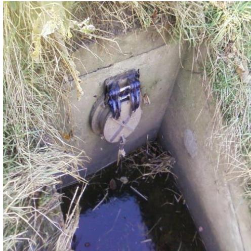
Figure 4.1: Photograph of a typical flap valve in Redbridge
