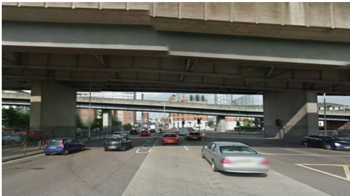
The junction underneath the A406 north circular flyover between Ilford and Manor Park.
