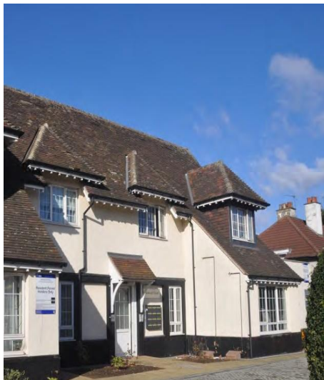
Hawbush Court - Housing conversion
