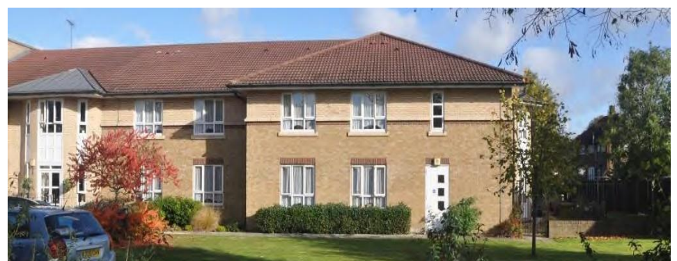
Chadwell House Residential Care Home
