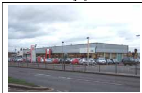
unsuitable structure in visually sensitive location
