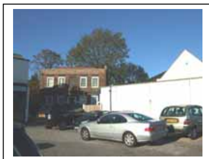
inappropriate setting and use of space
