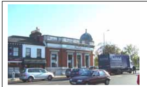
1920s former bank building
