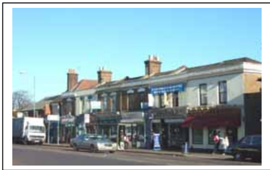
some inappropriate shopfronts & advertisements
