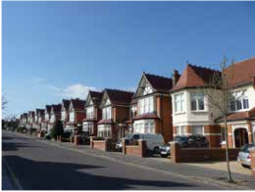
Fig. 41: Dramatic roofscapes and gables along Queen's Avenue, looking west
