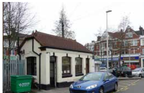
Fig. 47: Taxi office opposite Woodford Broadway Station
