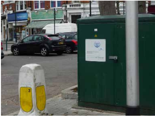
Fig. 33: Cable box within the station car park with bollard and streetlamp
