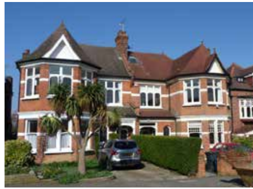
Fig. 42: Typical semi-detached pair showing decorative window joinery, Queen's Avenue
