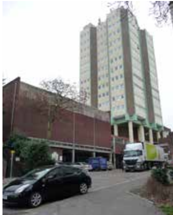
Fig. 21. View from Charteris Road on southern boundary of conservation area looking west towards service area rear of shopping parade (negative)
