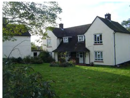
1. View showing the later south-western wing to Thurlby House
