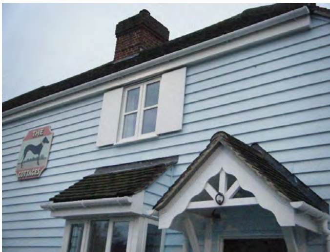
L. The locally listed 18 th century weather-boarded two-storey Greyhound Cottage is a key road frontage building within the Woodford Bridge Conservation Area
