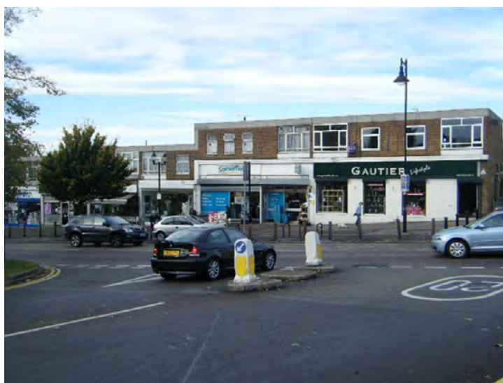
An example of modern obtrusive development within Woodford Bridge Conservation Area
