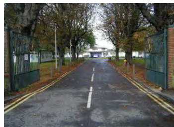
1 & 2. View of the sports pavilion building, and the tree lined approach to it
