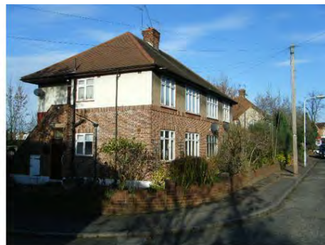
1, 2 & 4. Images showing the fine detailing the principal elevations of the Oakwood Close houses
