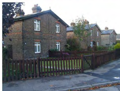
3 This large block (5-12 Cross Road) is particularly intrusive in the Conservation Area street scene
