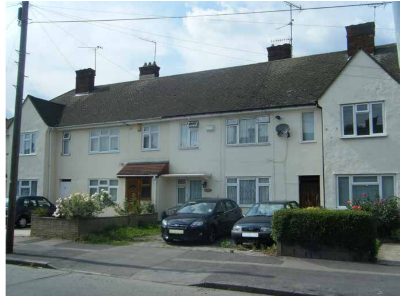
A suburban terrace east of Woodford Station. Note uniformity of composition and architectural simplicity.
