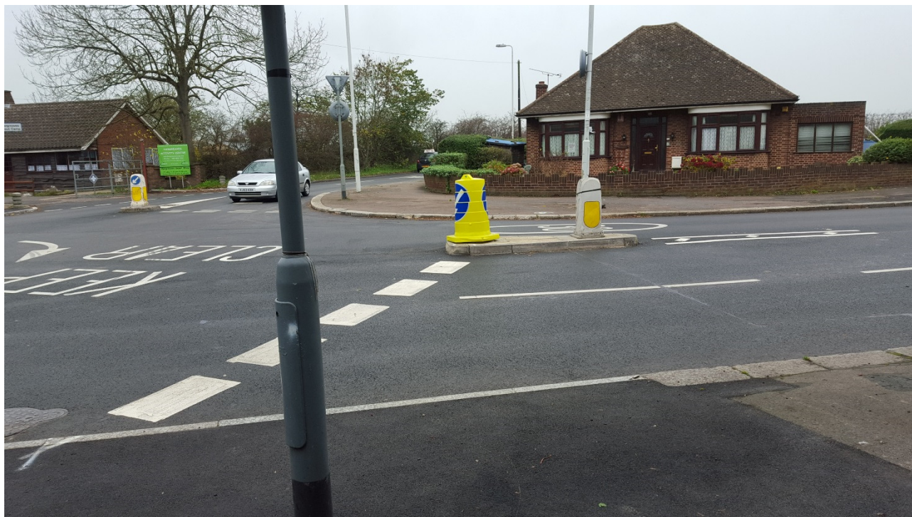
Figure 2-3 Junction of Billet Road and Hainault Road: Lack of Dropped Kerbs and Tactile Material
