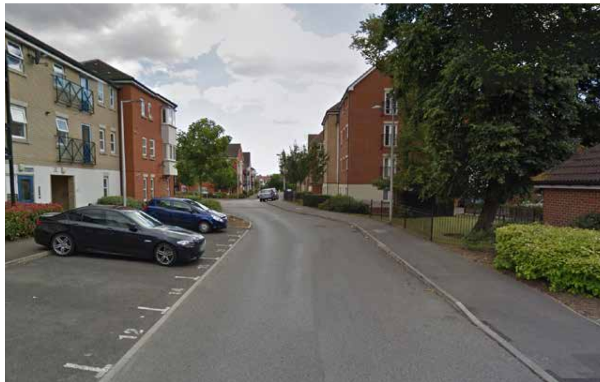
Figure 50 Taller buildings within Glandford Way
