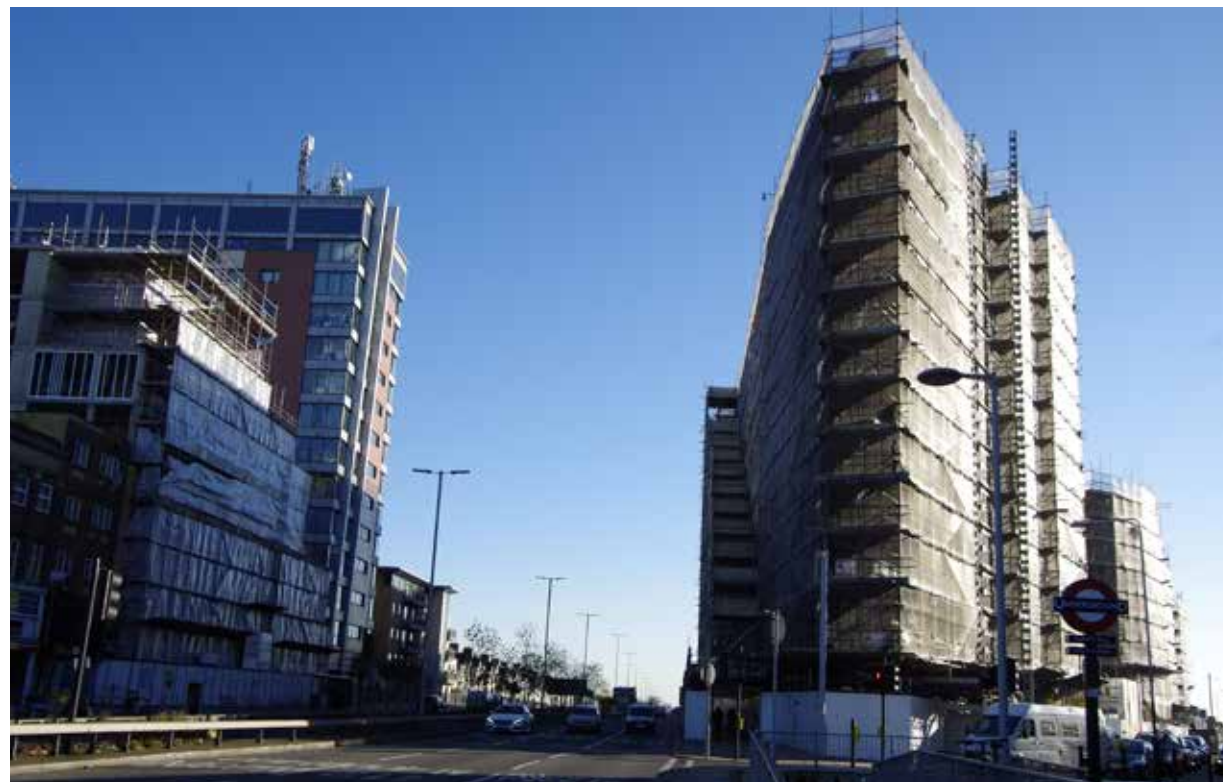
Figure 43 New development in the District Centre
