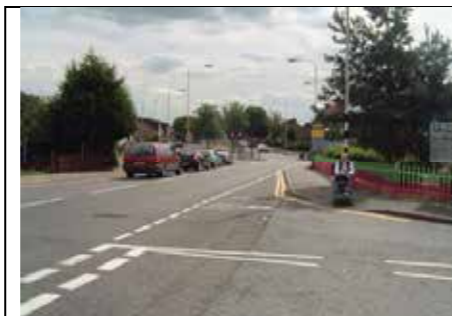
Wide entrance/exit splays to Station Road car park. Potential for conflict between vehicles/pedestrians.
