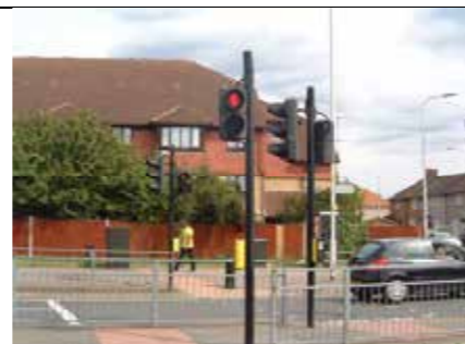
Poorly designed pedestrian/cyclist facilities at junction with Valence Avenue.
