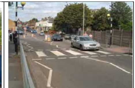
Pedestrian crossing located away from main pedestrian desire line. Poor road layout at junction beyond.
