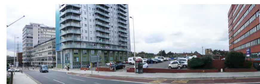
Iford Hill, towards Western station Entrance
