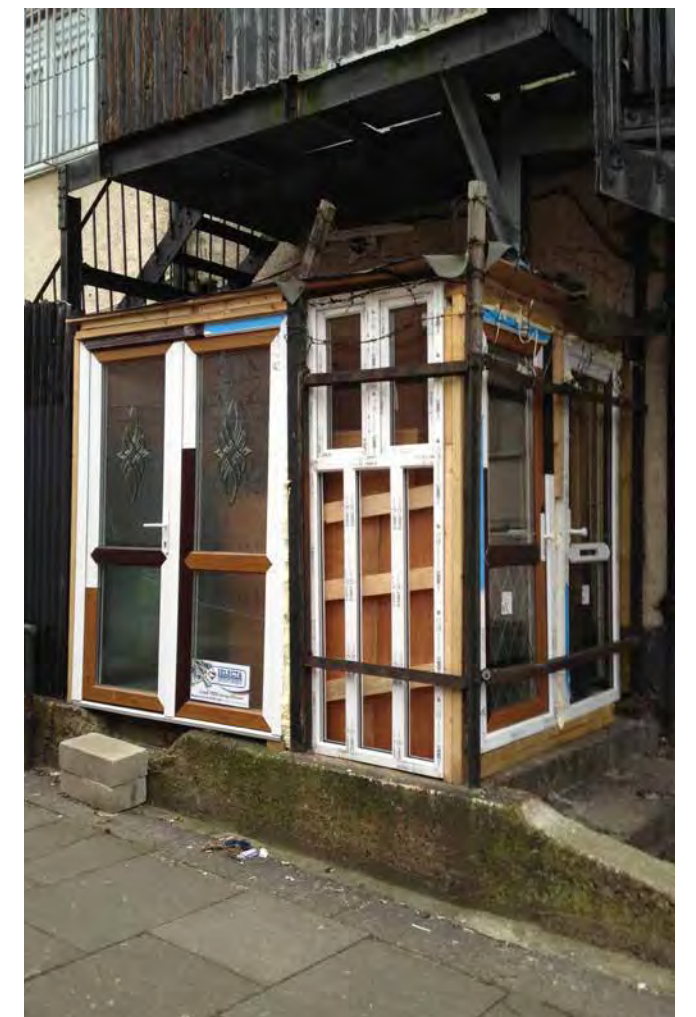
11 - Further image of the back of house on Salisbury Road.
