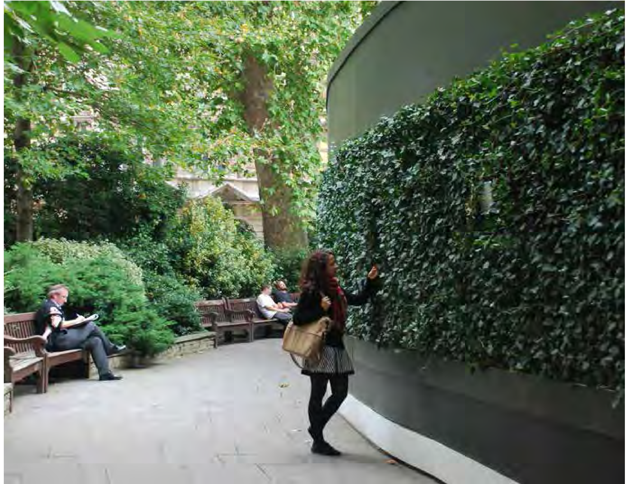
Crossrail installed green wall around worksite at Finsbury Green, City of London
