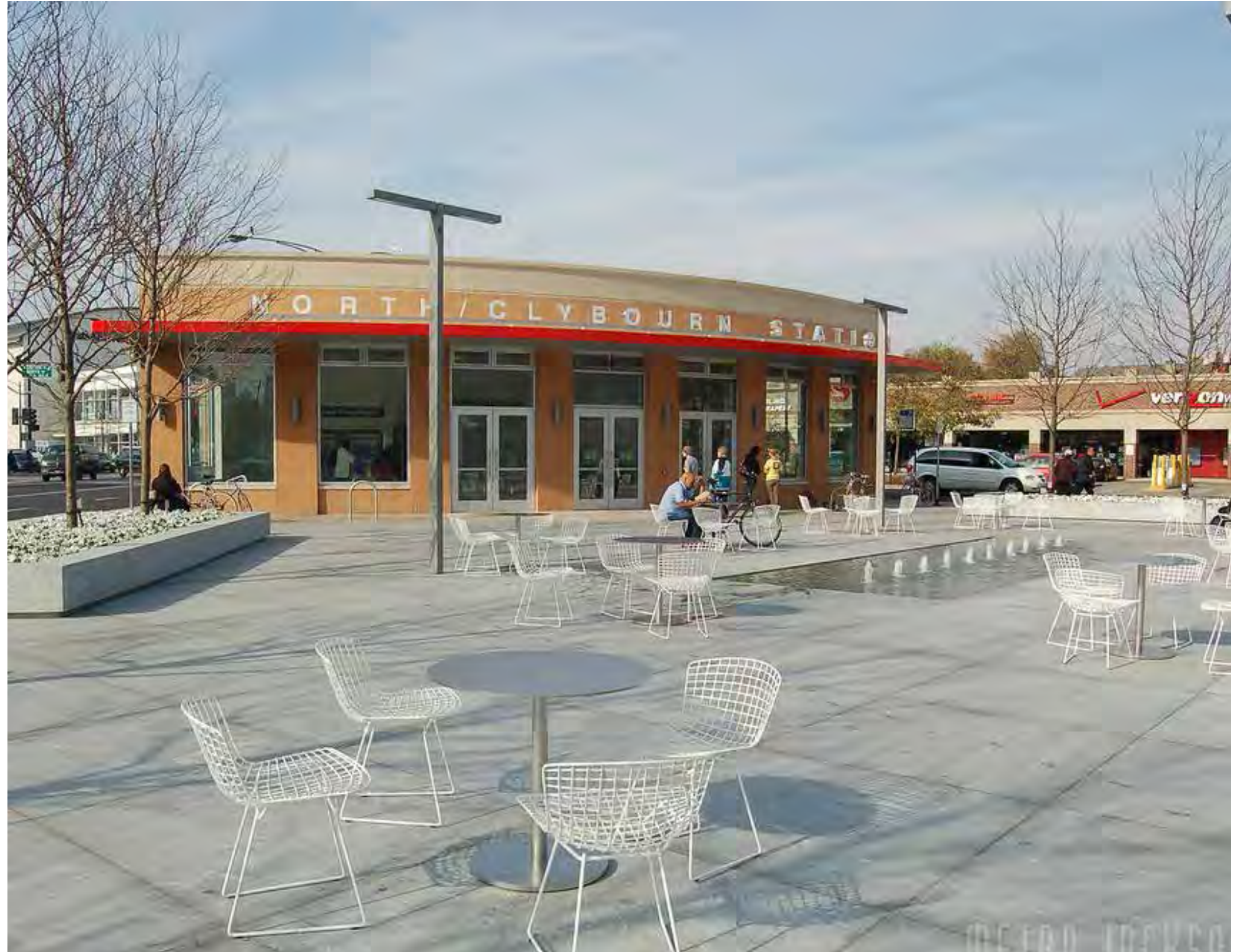
North Clybourn Station, Chicago
