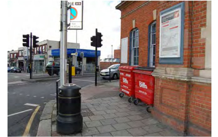
12 - Large refuse bins located at front of station and on the pedestrian footway. Detract from the visual amenity of the area. .
