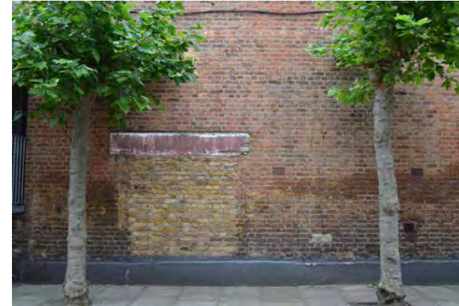
7 - A further example of the blank elevations dominating Farley Drive's boundaries.
