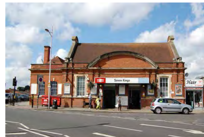
11 - Seven Kings Station - main entrance .
