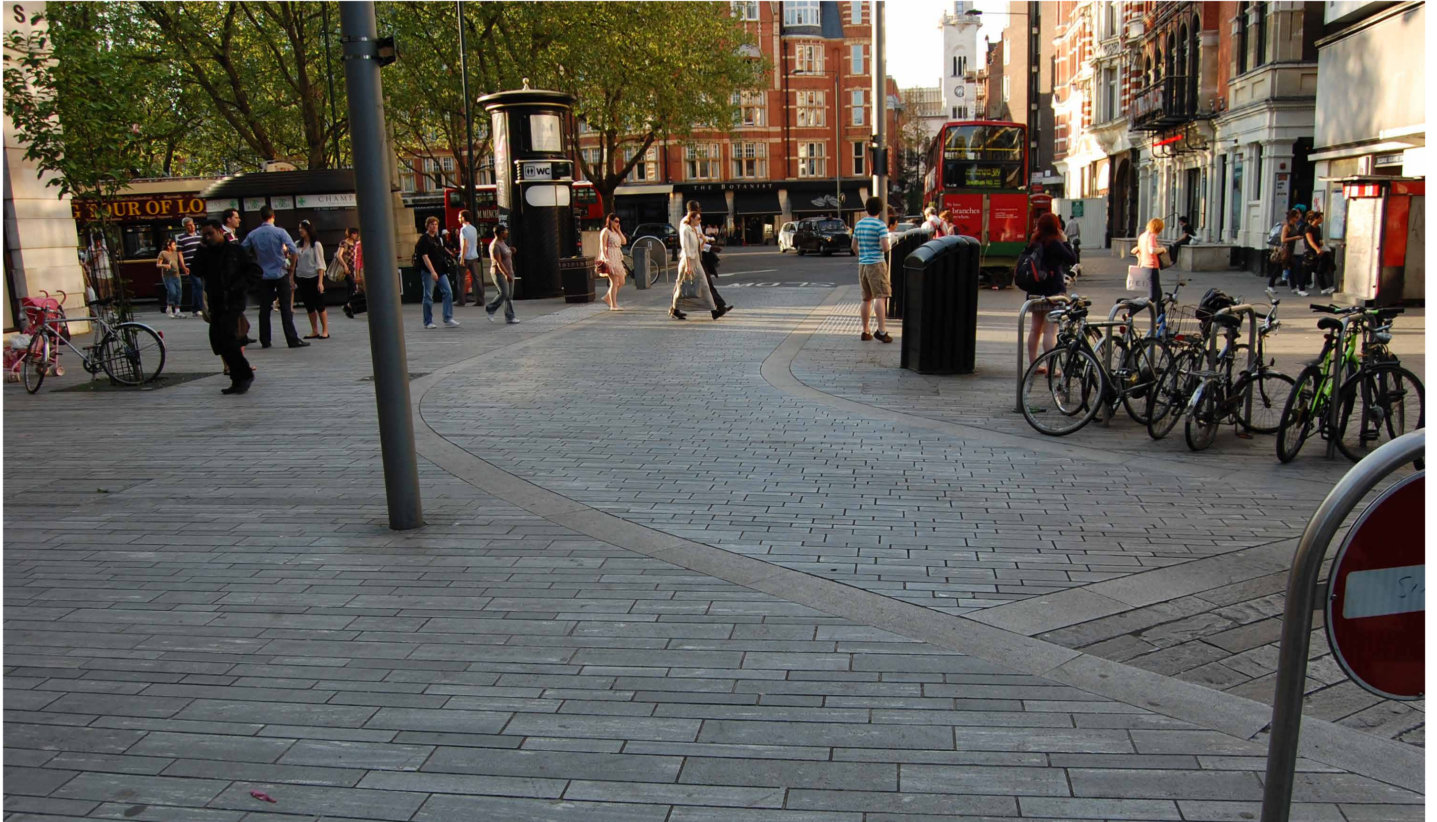
Holbein Place level crossing to front of Sloane Square underground station. Single granite sett surface.
