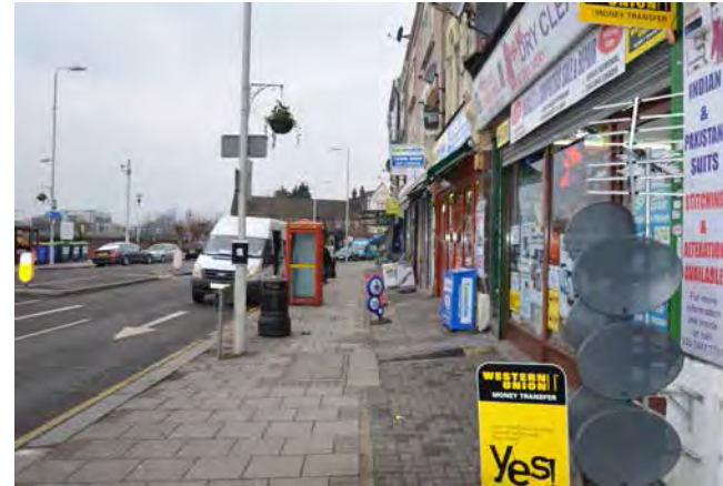
2 - Poor shop forecourt connections to pedestrian footway. Additionally there is an excess of un-aesthetically pleasing street clutter.
