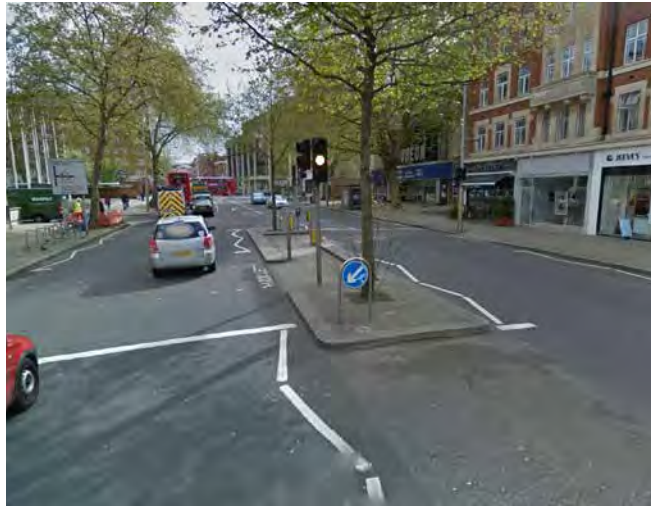
Staggered pedestrian crossing, with no railings
