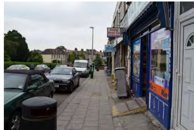
6 - Poor shop forecourt connections to pavement and avoidable, un-sightly clutter.
