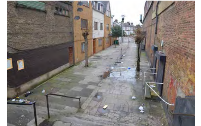
8 - It is evident from the ponding that the drainage could be improved. The broken paving and litter suggest a space that is neglected and unloved.
