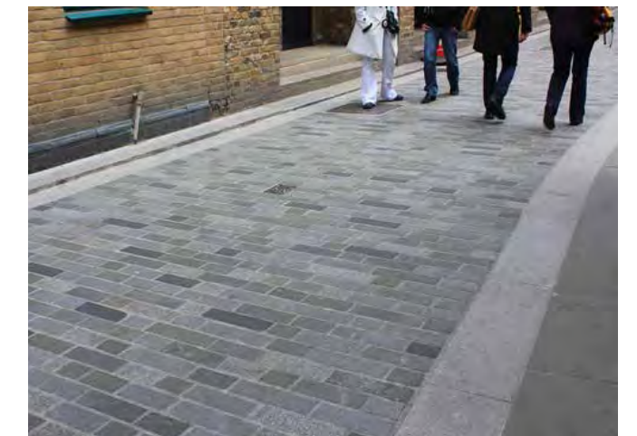
Example of granite sett carriageway surfaces
