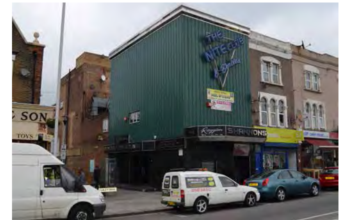
12 - This ugly building extends back to define the eastern side of Farley Drive and its redevelopment offers the potential to animate the route.
