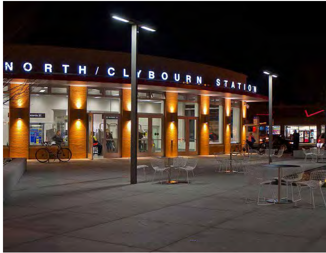
North Clybourn Station, Chicago, at night
