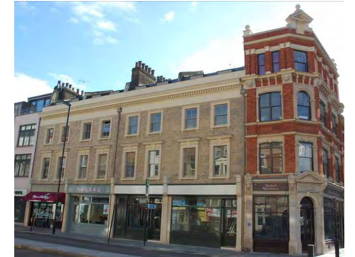
High Street, Whit Chapel renovations - after
