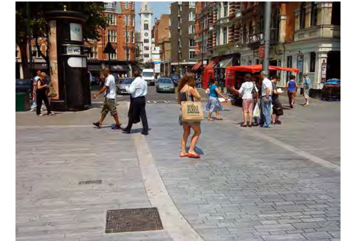
Example of granite sett carriageway surfaces
