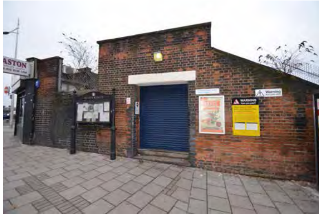
1 - Secondary station entrance in Cameron Road.
