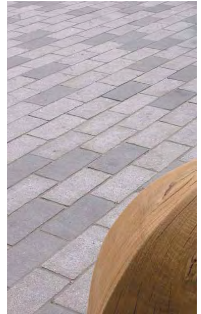
Granite setts surface for raised crossing table
