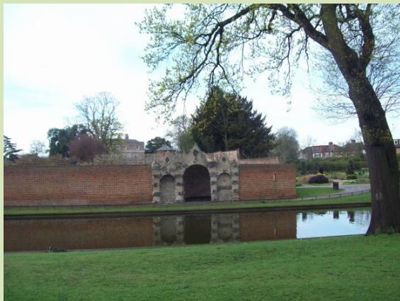
Restored heritage features at Valentines Park (a quality exemplar site)
