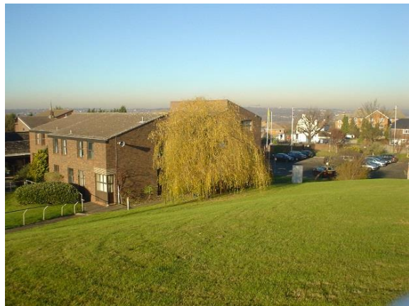
Existing admin and accommodation block
