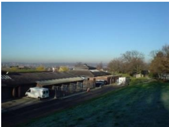
Existing kennels in the Green Belt
