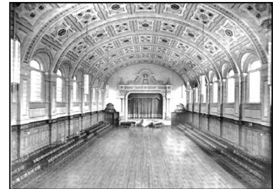
Recreation hall interior (c1960)
