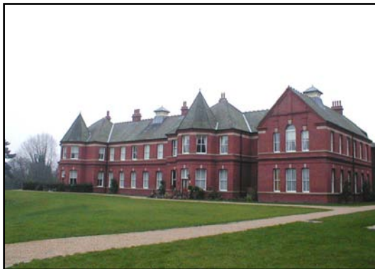
Two-storey ward block
