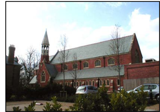
Former chapel, eastern elevation
