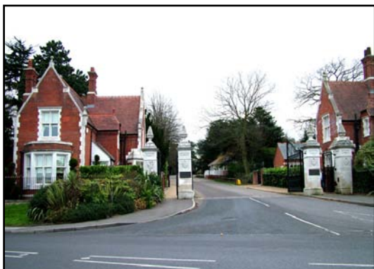
Entrance lodges & gate piers on Manor Road
