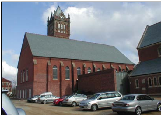
Former recreational hall and water tower
