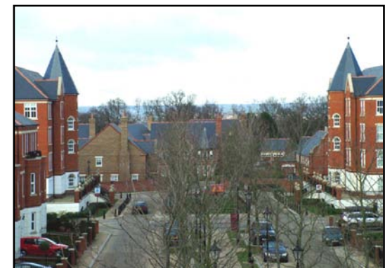
Infill boulevard development
