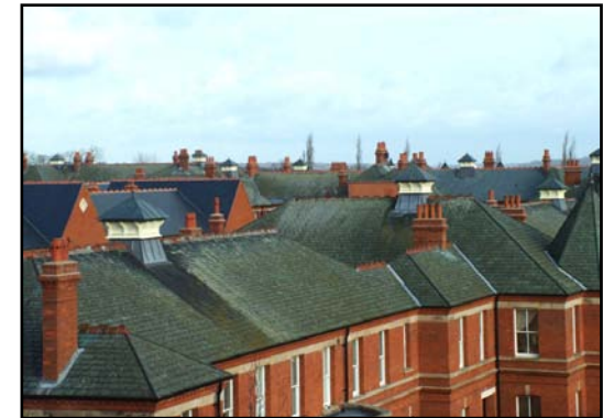
Roofscape of former hospital
