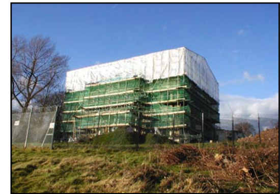
Claybury Hall - during restoration
