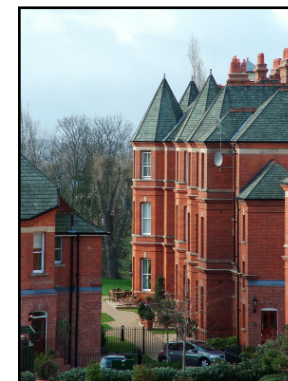
Projecting tower with vaulted roof
