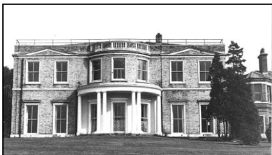
Claybury Hall - front elevation (c1970)
