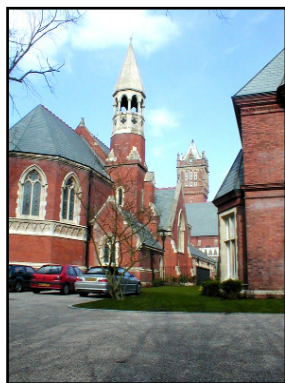
Former hospital chapel & water tower
