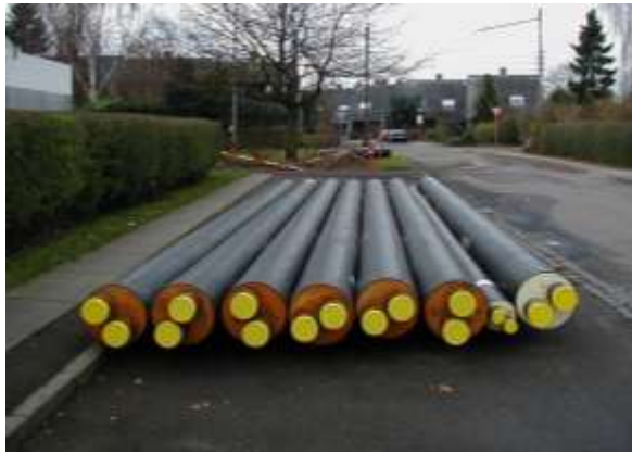
Figure 40: Twin Pipes for District Heating (image courtesy of Ramboll)
