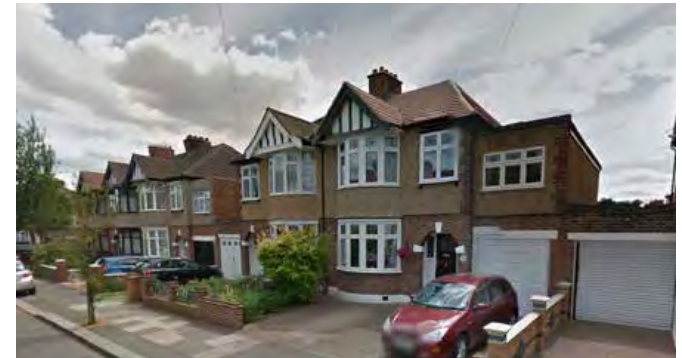
Figure 19: Post-war terraced Housing on Priestly Gardens
