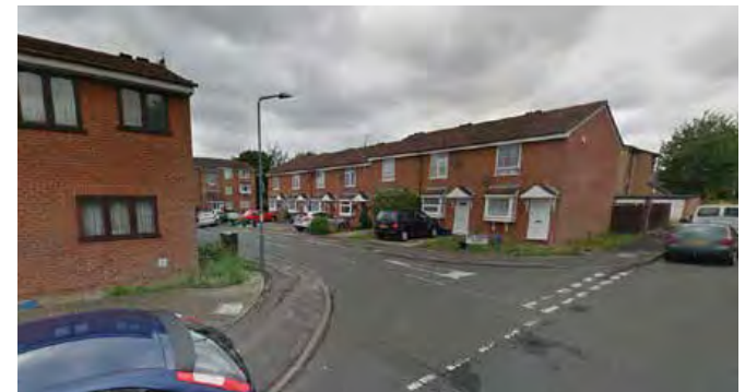
Figure 20: Poor quality 1980s terrace development at Millhaven Close
