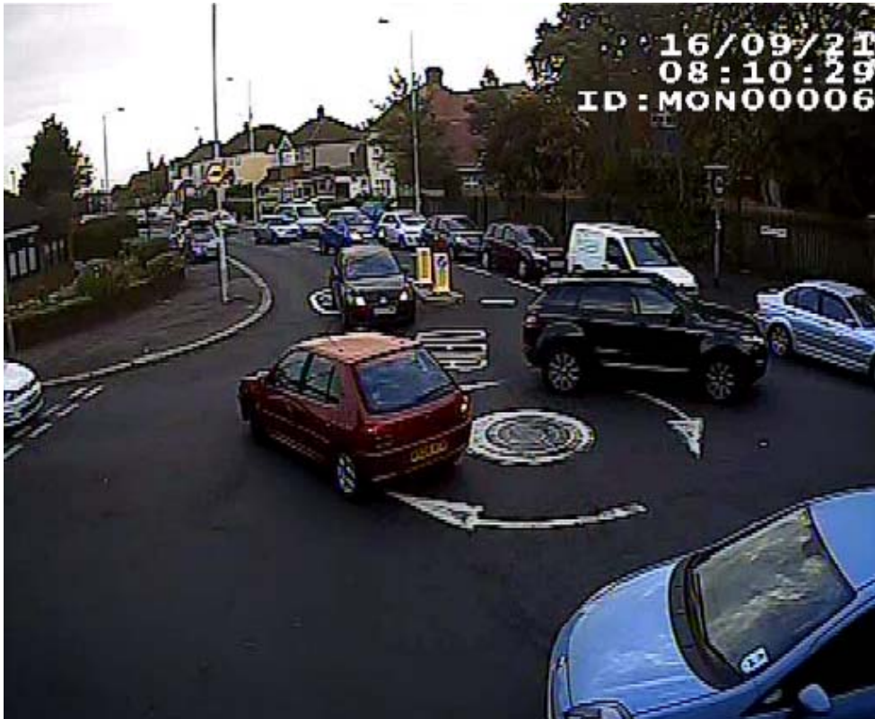
It should be noted that the second westbound lane is only 30 meters long, starts at the first lamp post on the right of the picture, vehicles turning right travel along the wrong side of Billet Road creating a pinch point for eastbound traffic.
