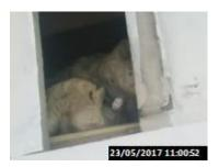
Observation: Exposed wiring was identified that was not properly isolated and capped off. It could not be confirmed whether this wiring was still live.
